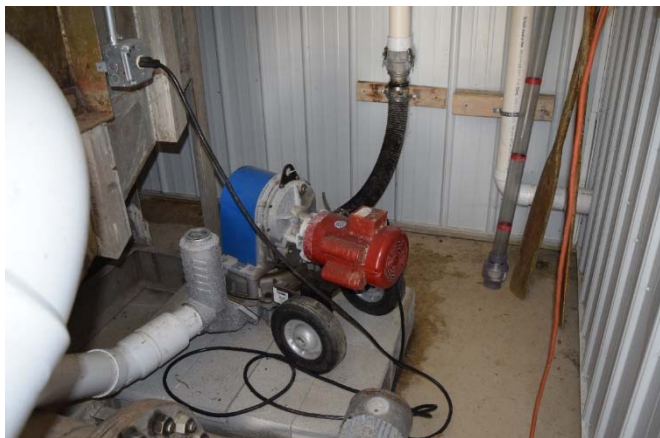
Pumping Algae Sludge to Geotube®
