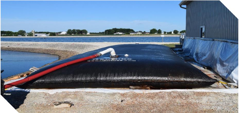
*Geotextile tube container in place to accept slurry to capture iron sediment and allow filtrate water to escape back to the lagoon.*
