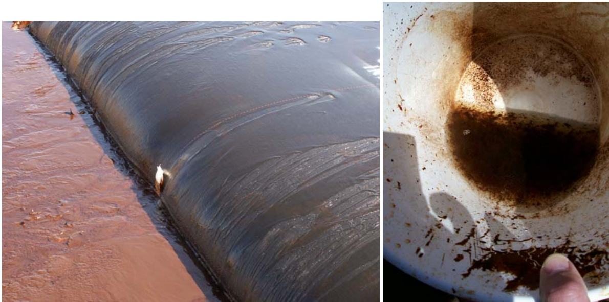
Figure 8 – Clean filtrate from the Geotube® containers was discharged from the equalization basins via the sand filters.
