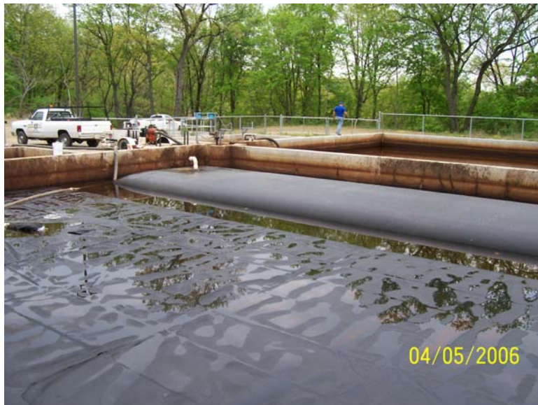
Figure 4 – A 30-ft circumference x 72-ft long Geotube® and a 45-ft circumference x 100-ft long Geotube® were installed in the north equalization basin to contain and dewater approximately five hundred thousand gallons of residuals accumulated in the south basin.
