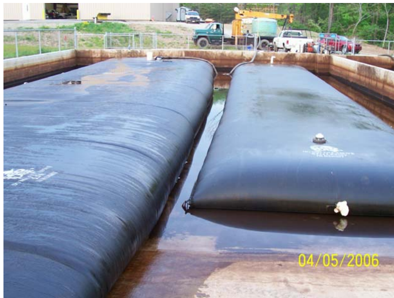
Figure 6 – A 30-ft circumference x 72-ft long Geotube® was pumped to 75% capacity (right) and filling of a 45-ft circumference x 100-ft long Geotube® (left) was initiated for back-wash residual dewatering and consolidation.
